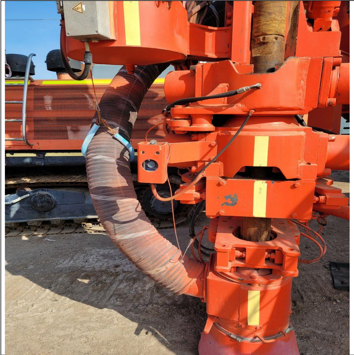
Break table and rod holder in good condition
