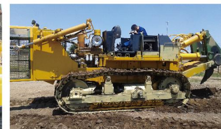
推土机现场大修服务 Bulldozer repair services
